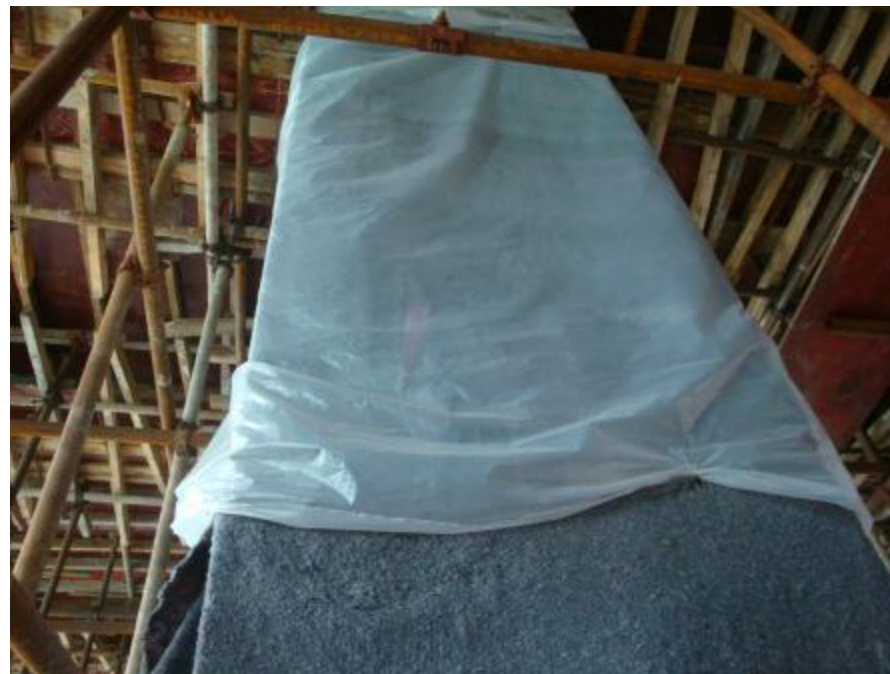
拆模后养护龄期内覆膜养护
